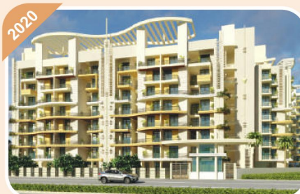
SAI DHAM RESIDENCY Adjacent BHS, Civil Lines, Prayagraj
