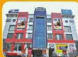
P SQUARE MALL Civil Lines
